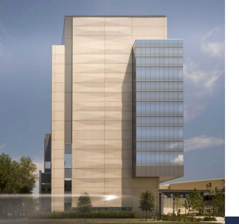
The undulating precast concrete façades use light, reflection, and shadow to catch the sun as it plays across each building's surface....
